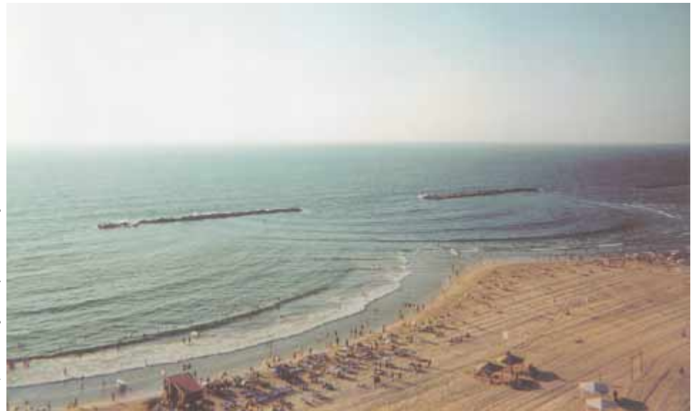
At a beach in Tel Aviv, Israel, plane water waves pass through two openings in a breakwall. Notice the diffraction effect—the waves exit the openings with circular wave fronts, as in Figure 37.1b. Notice also how the beach has been shaped by the circular wave fronts.
